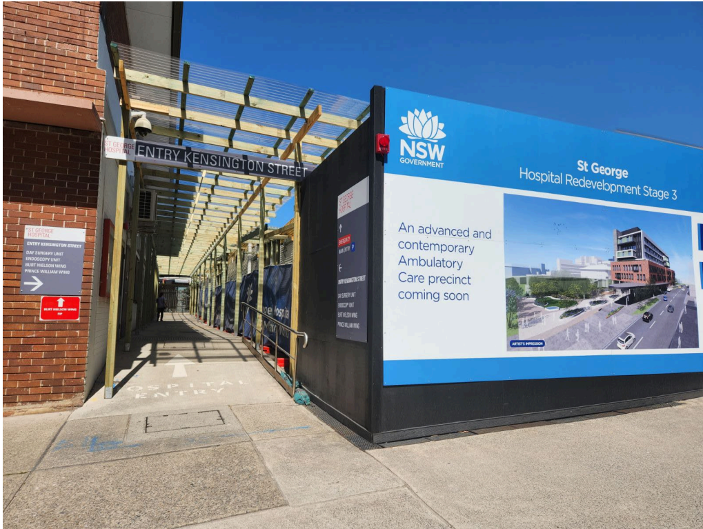
Kensington Street - Pedestrian Entrance
